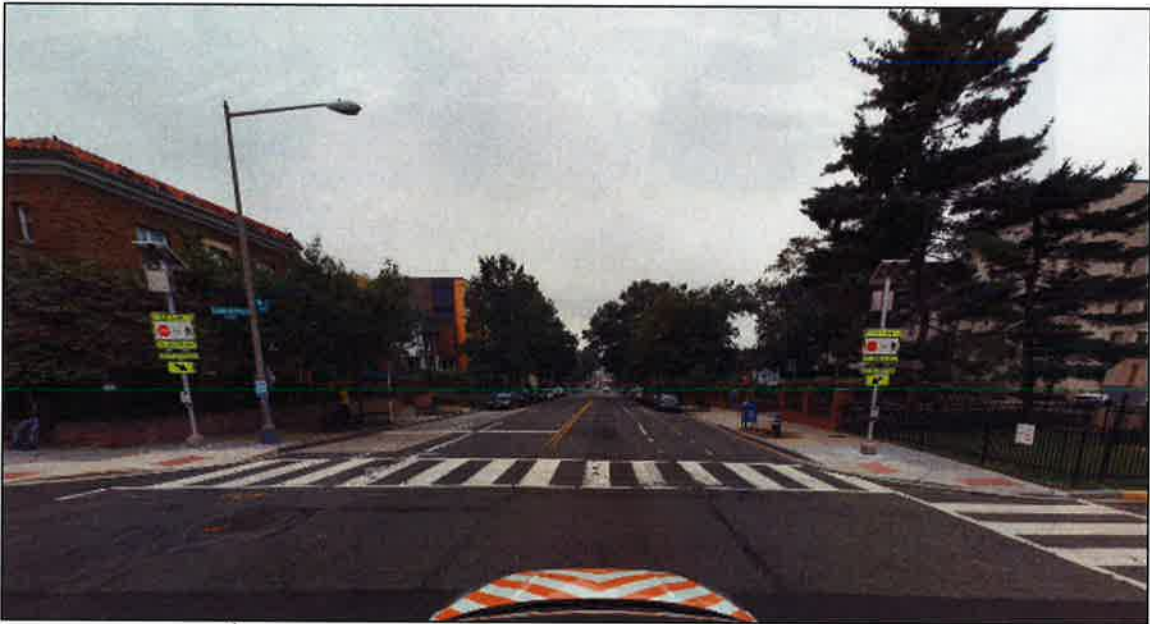
Figure: RRFB – 14 th Street at Randolph Street NW
